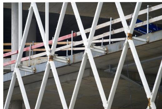
FIG. 3 The diagonal grid of the façade of MyZeil shopping centre in Frankfurt am Main (by architect M. Fuksas, 2009). The façade smoothly transforms into the triangulated geometry of the free-form roof. The figure shows the sub-structure of the façade grid attached to the floor slabs before the façade profiles were mounted.
