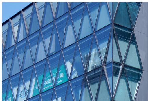
FIG. 2 J6 Front in Tokyo Omotesando (by architect Matsuda Hirata Design Inc., 2008) features a diagrid of structural supporting elements with a diagonal grid of façade elements.
