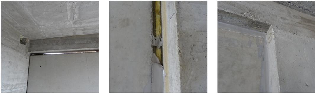
FIG. 7 Sealing joints of panel and load-bearing structure
