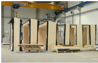
FIG. 12 completed modules in factory
