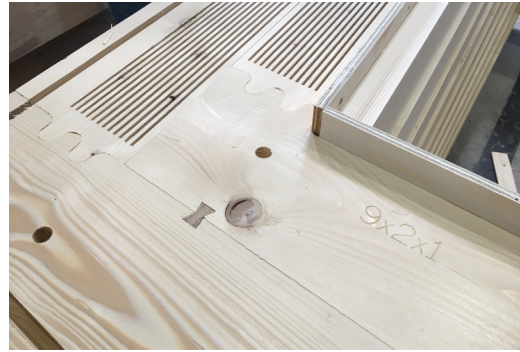
FIG. 11 Assembled corner lap joint detail
