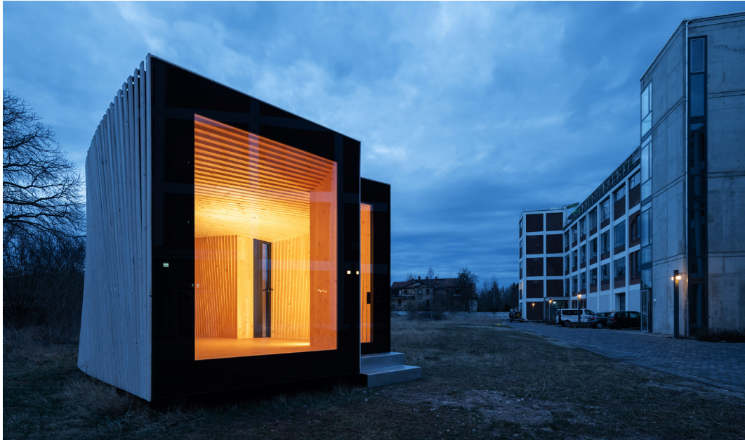
FIG. 15 Completed IBA: Timber Prototype House Demonstrator
