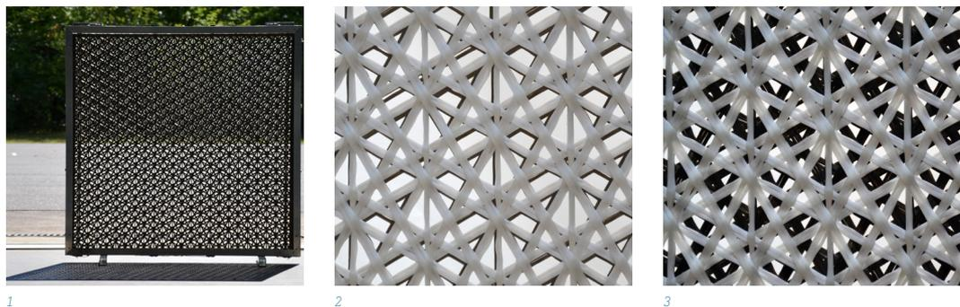
FIG. 6 Demonstrator of ADAPTEX Mesh within the constructional frame (1) facing the inner surface; close-up of open state (2) and close-up of closed state (3) facing the outer surface
