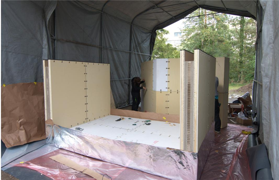
FIG. 9 Floor and wall modules. Assembly of the roof in the background
