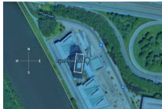
FIG. 14 Aerial view of the Westraven building, showing aspect.
