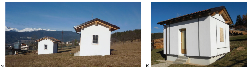
FIG. 10 Test cell A, in the background, and test cell B before retrofit (a); test cell A after retrofit (b).
