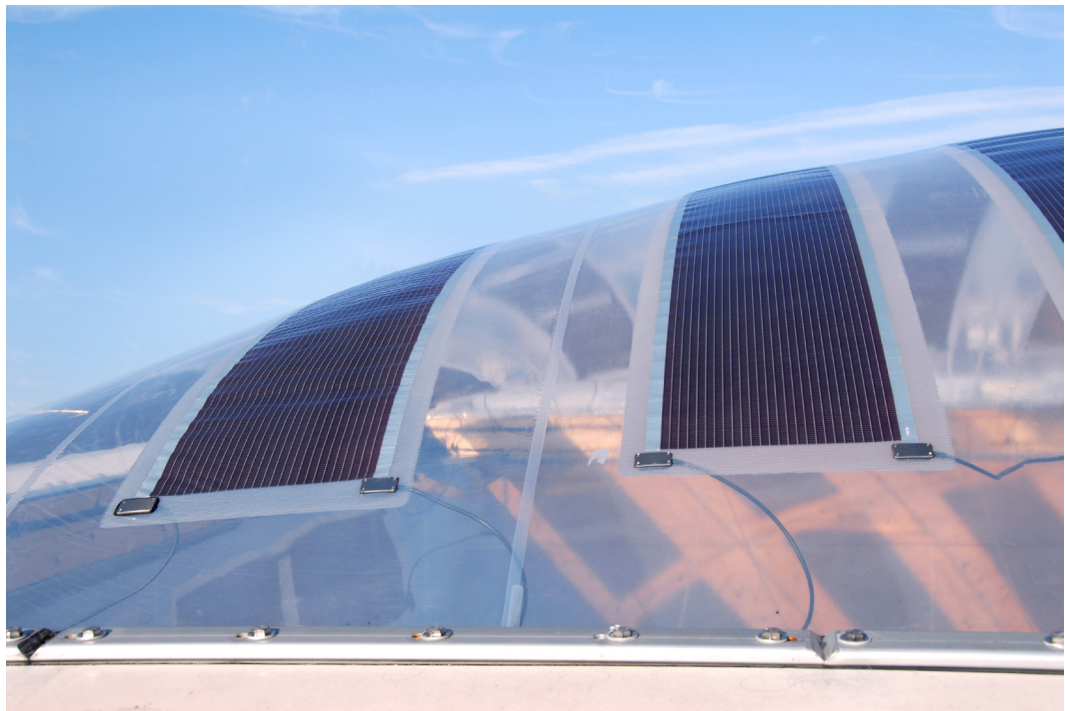
FIG. 7 PV laminated to structural ETFE top layer of a cushion (source: author)
