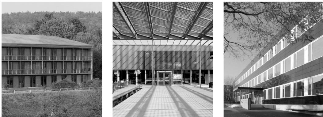
FIG. 1 Non-structural BIPV with modules as roof covering (left) and structural application as roof glazing or façade glazing. ©Marché International, Kempthal/CH (left), Bruno Klomfar (middle), Stefanie Flohr, TU Dresden (right)
