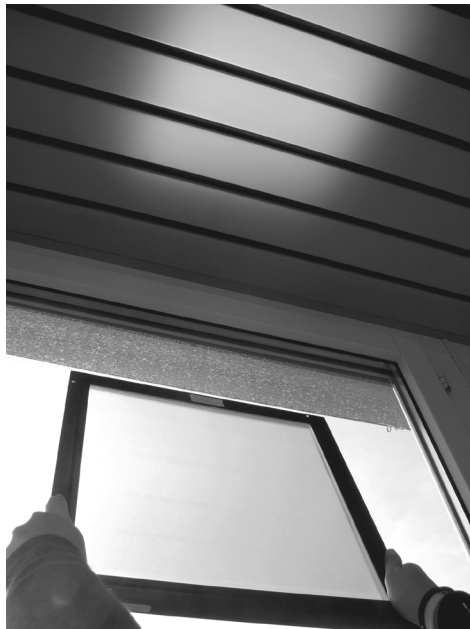
FIG. 1 DRC_1 deflecting sunlight upward
