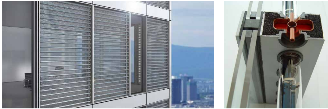
FIG. 2 Left. Vacuum pipe collectors integrated into a modular curtain wall providing a glazed façade. Right. Detail of the prototype (University of Stuttgart, n.d.)
