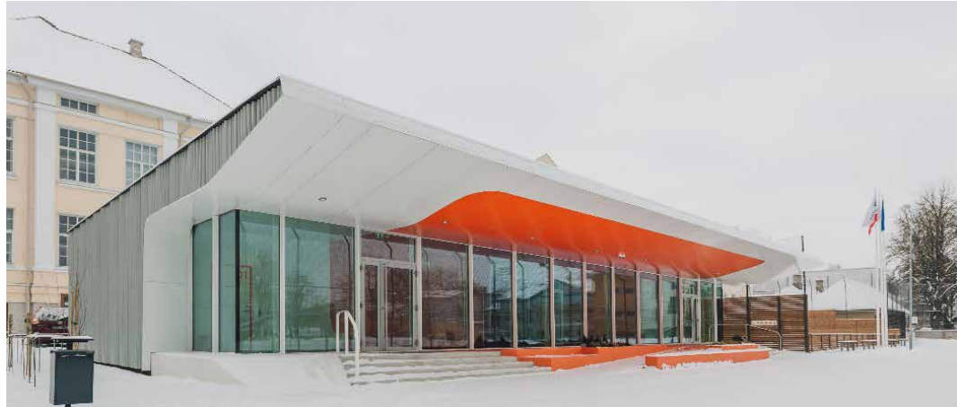
FIG. 8 External view of the Tartu demo building. The front curtain wall was developed through the Osirys project like the rest of the façades (which use the multilayer façade solution). The partitions inside the building also use the Osirys developments.
