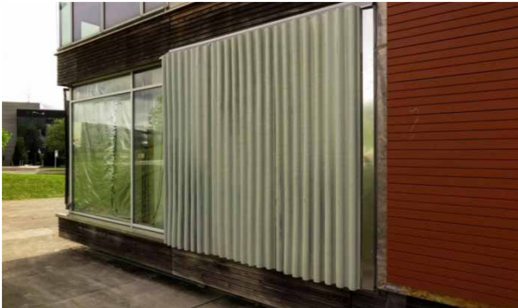
FIG. 6 Multilayer façade installed in Kubik test cell
