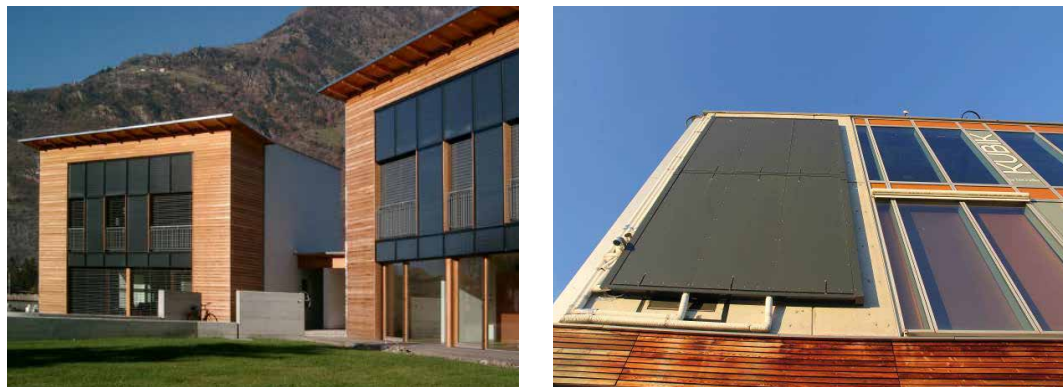
FIG. 1 Left. Glazed flat plate collector integrated into a modular façade system (Winkler Solar, n.d.), Right. Prototype of unglazed collector integrated into a metal cladding panel (Elguezabal, Garay & Martin, 2017).
