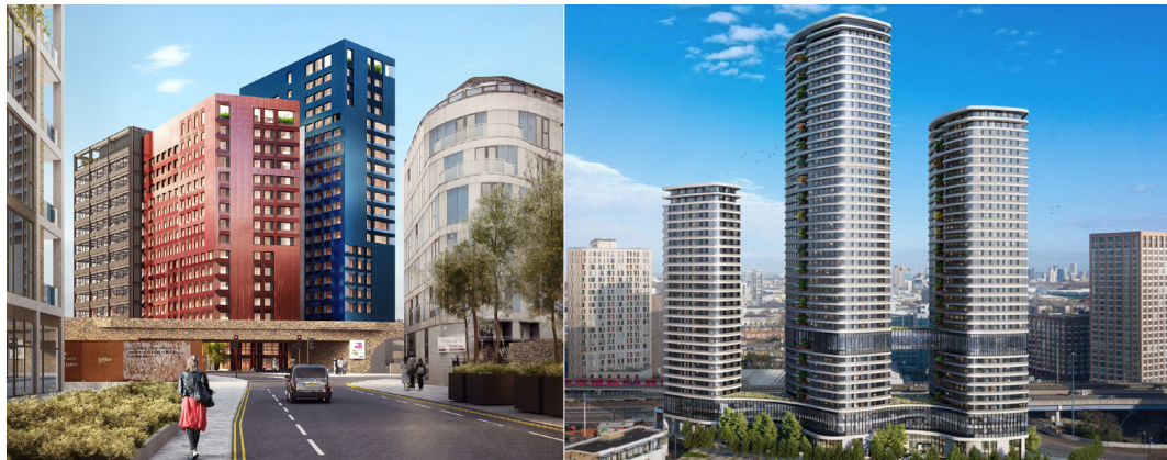
FIG. 3 Render images of the two projects used to test the automated process. Courtesy of Alford Hall Monaghan Morris, Apt and Urbanest.
