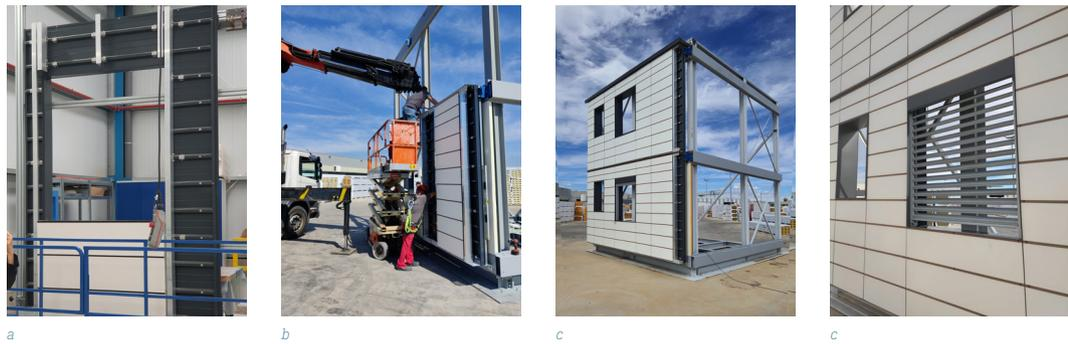
FIG. 10 Demonstration prototype: a) Assembly of TPP in the PnP using a vertical working station; b) Movement of the PnP module using a crane; c) Final asset of the prototype; d) Detail of window and sun shading integration.
