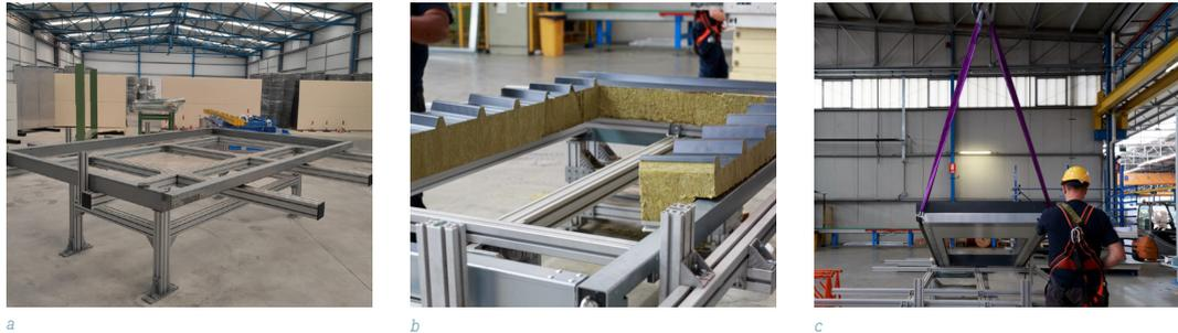
FIG. 8 Preliminary prototype: a) LSF structure on horizontal working station; b) Assembling the PnP module on the horizontal working station; c) Lifting of the module vertically once preassembled.
