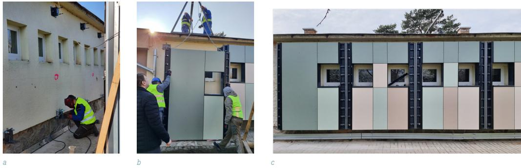
FIG. 11 Final prototype: a) Placement of the anchoring system on the existing building structure; b) Transportation and installation of the PnP module; c) Final façade configuration after the renovation with the PnP module.
