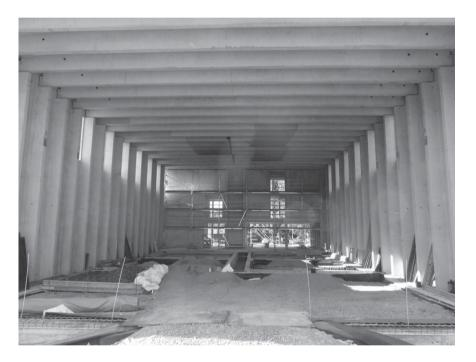
Fig. 10. Interior view of the rib structure of the industrial hall.
